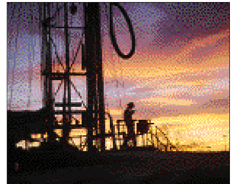
A driller installs a public water-supply well in Scottsdale, Ariz.
